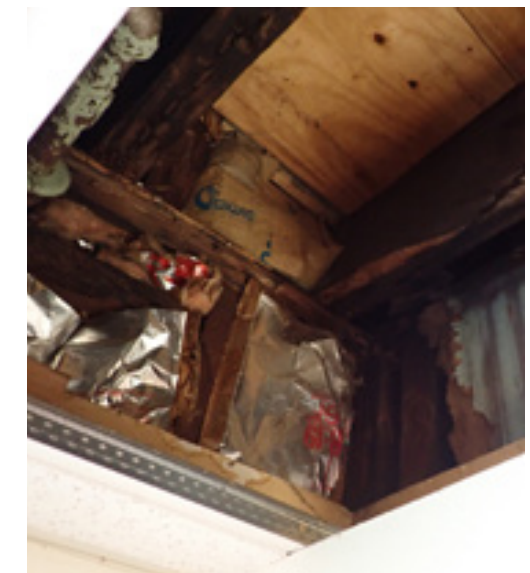
Ceiling Above Main Entry, July 2019
