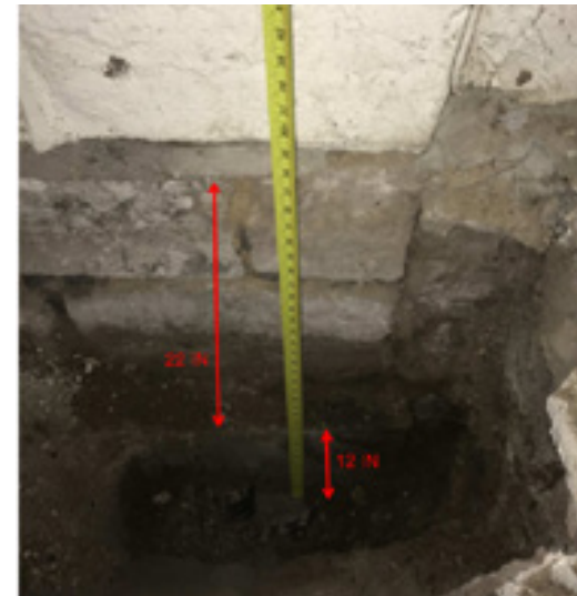
Test Pit TP-1, Footing 20" Below Grade, Geotechnical Report, September 2019
