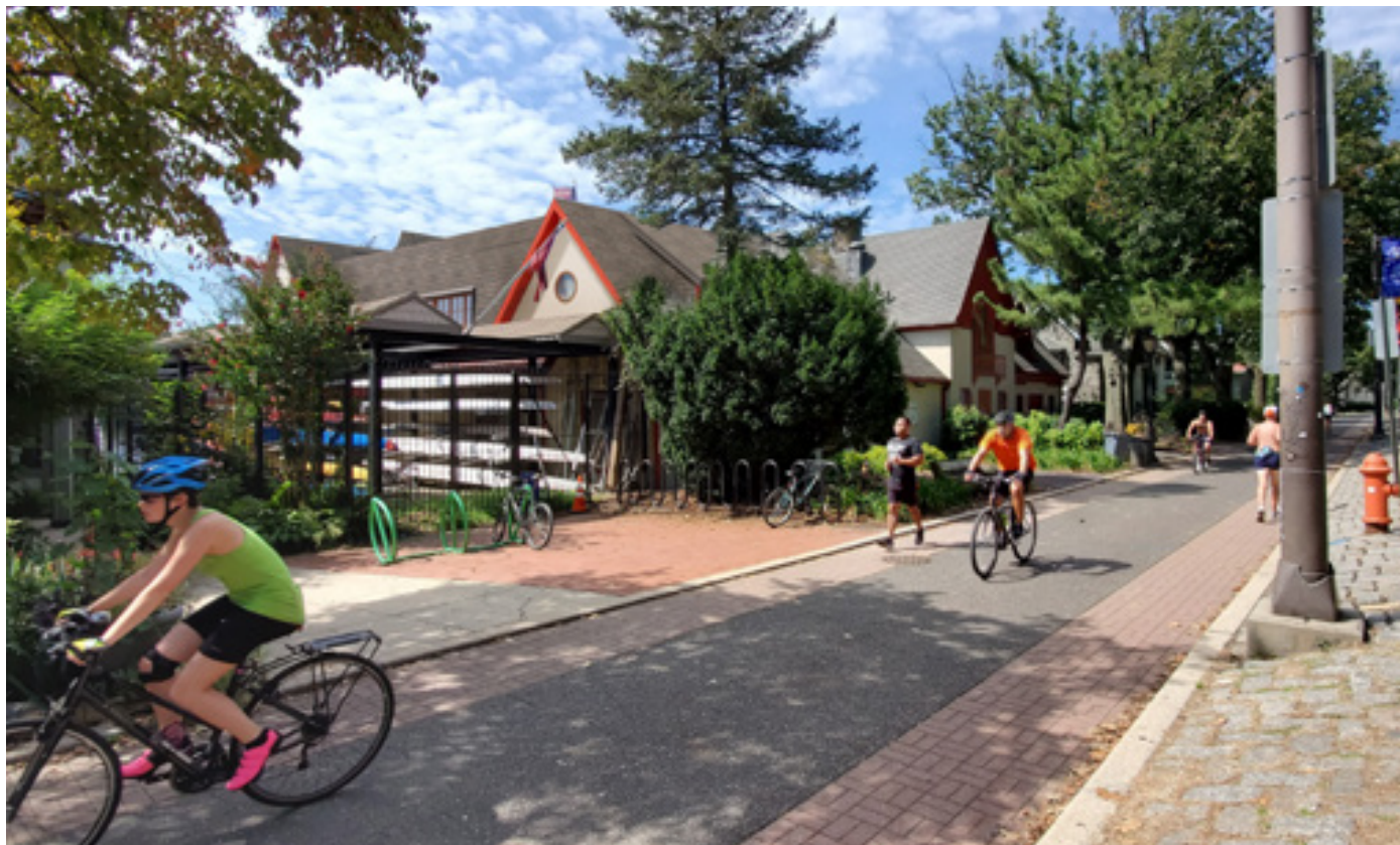
View of the East Elevation from Kelly Drive
