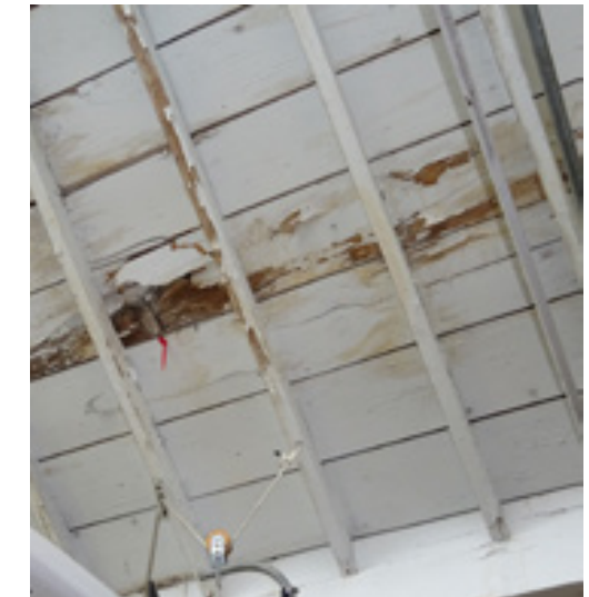
Roof Above Men's Boat Bay, July 2019
