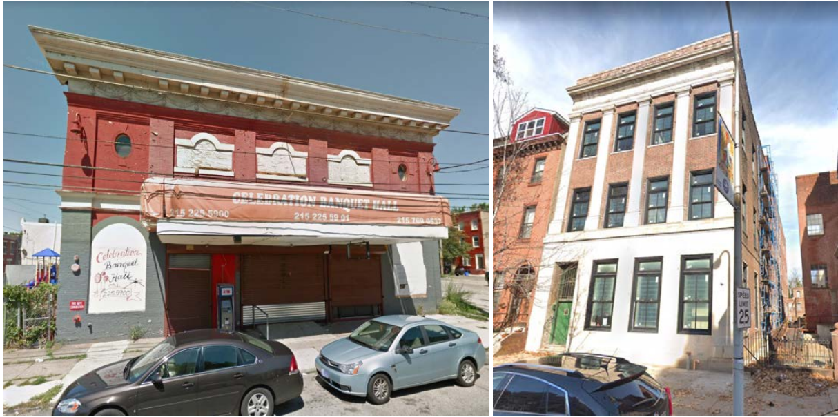
Figure 20. (Left) Liederkrantz Hall at 2709 Cecil B. Moore Avenue. (Right) Improved Order of Redmen clubhouse at 1521 W Girard Avenue. (Source: Google Street View)
