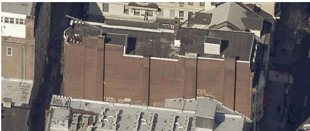
Figure 8: East elevation from Walnut Street (Top; source: Cyclomedia, 2019); Birdseye view of east elevation (Bottom; source: Pictometry, 2019)
