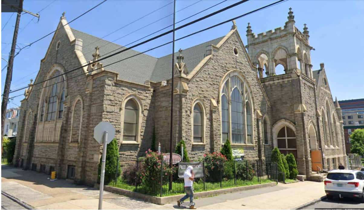
Figure 22. Nativity Lutheran Church and Rectory at 3501-05 N 17 th Street. (Source: Google Street View)
