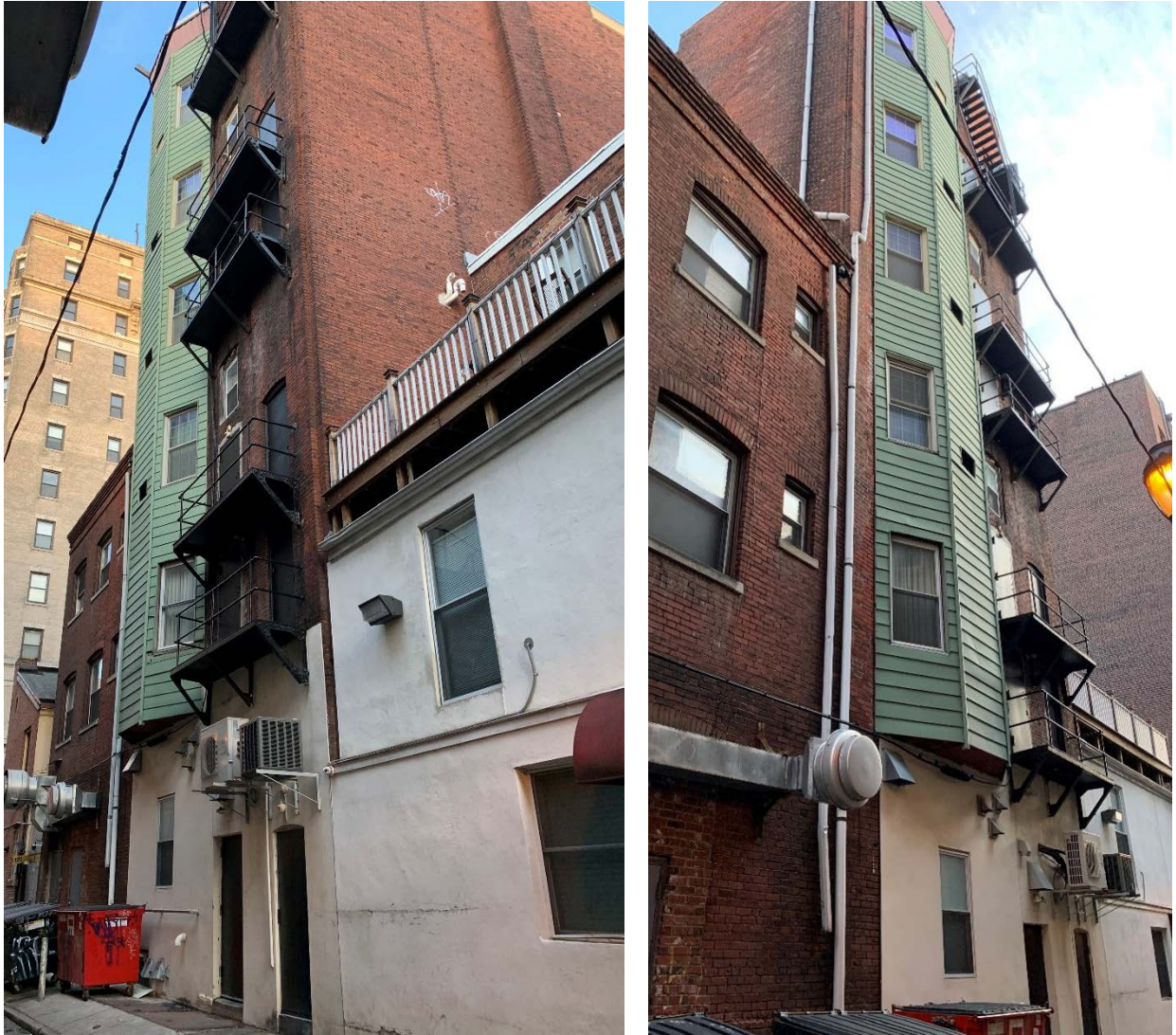
Figure 9. Rear elevation on Chancellor Street, January 2020. (Source: Philadelphia Historical Commission)
