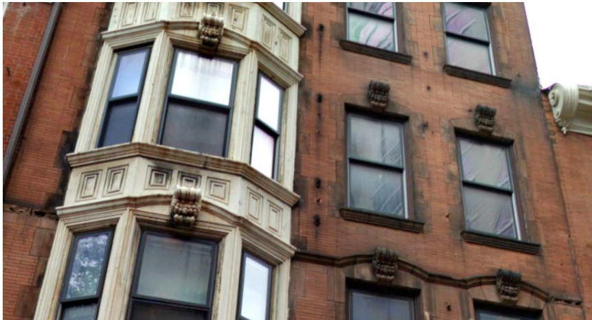
Figure 5: North elevation details, floors 2-5, 2019. (Source: Cyclomedia)
