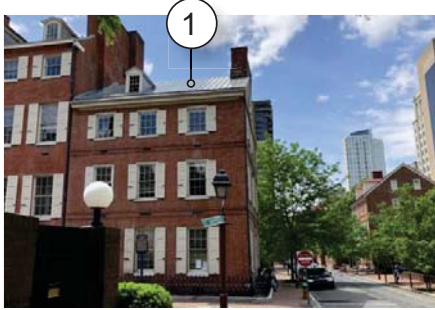
REFERENCE IMAGE - METAL ROOF
