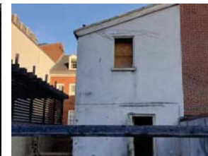
Leithgow Street upper facade. Image Dated: 05.15.2019
