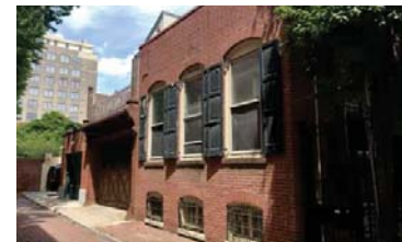
Leithgow Street looking at ground level existing buildings. Image Dated: 05.15.2019
