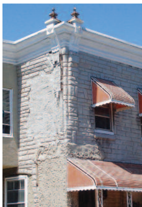
Left: Permastone and stucco cover original brick
