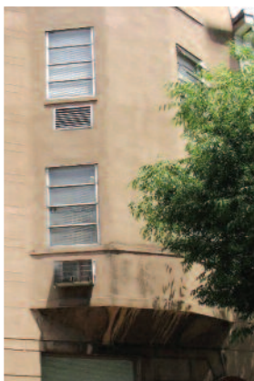
Left: Permastone and stucco cover original brick
