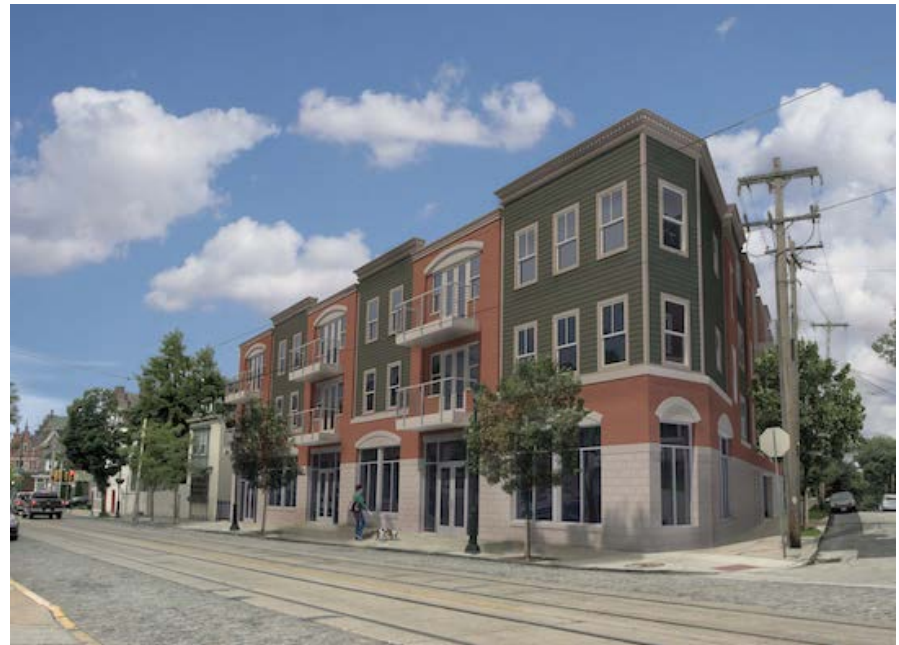
Figure 19: Mixed-Use Development (6600 block of Germantown Ave)
