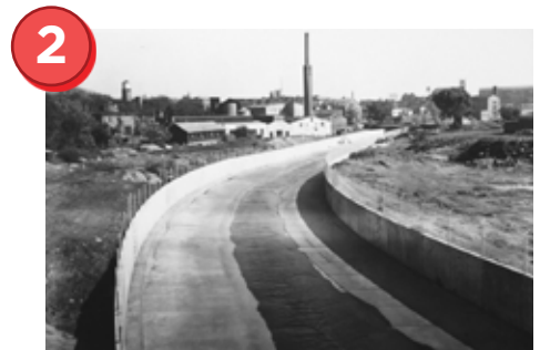
1950, Creek channelization between Castor Avenue and Wingohocking Street Source: City Archives of Philadelphia
