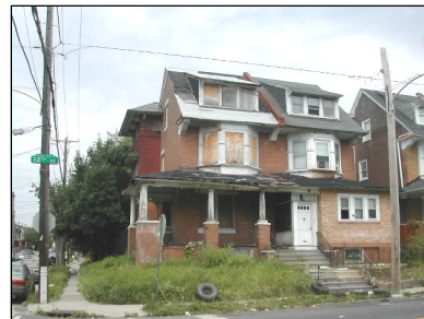
Corner home in need of major rehabilitation on 12 th Street.
