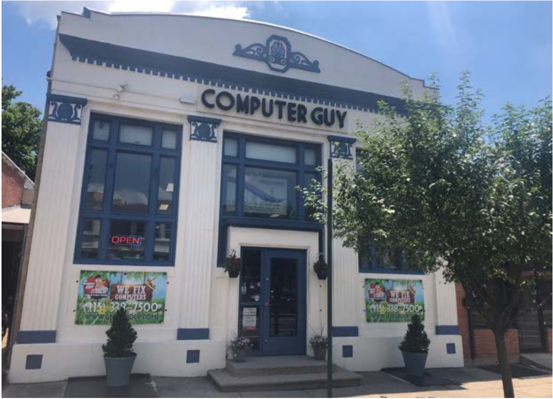
Figure 4. Front façade of 6911 Torresdale Avenue. Credit: Alex Balloon, 2018.
