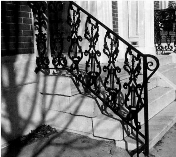
Masonry steps should be maintained to prevent the damaging effects of water penetration.
