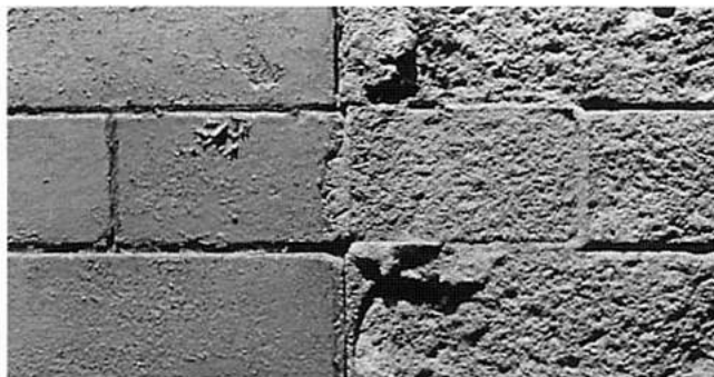
The negative effects of abrasive cleaning or sandblasting on brick are evident on the right.
