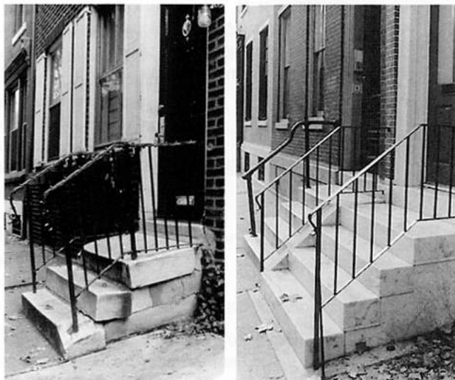
Masonry steps should be maintained to prevent the damaging effects of water penetration and subsequent freezing and thawing.
