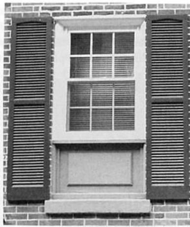
Left, preserve wooden windows and shutters. Right, an inappropriate window replacement.
