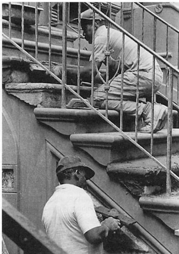
Masons applying a finish coat of stucco.
