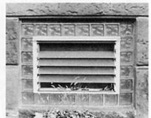
Original basement window grilles are part of the building's design; inappropriate alterations are jarring.
