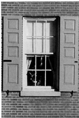
Left, preserve wooden windows and shutters. Right, an inappropriate window replacement.
