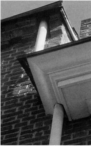
Pole gutters are a typical Society Hill feature. They should be kept intact and in good working order.
