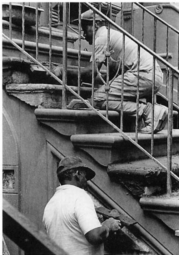
Masons applying a finish coat of stucco.
